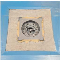
3. Install Grid Adapter into the drain and onto an solid bed of tile adhesive.
