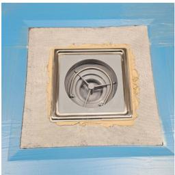
4. Apply tile adhesive to the inside of the PK155 Grid Frame.
