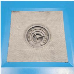
2. Ensure the Mini Drain Clamping Ring is seated correctly.
